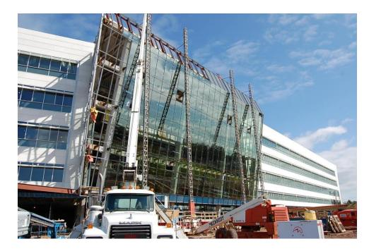
FIGURE 22: CURTAIN WALL CONSTRUCTION [TAKEN ON 10/4/2011 BY AL BATTEN, R.A. KENNEDY & SONS INC.]
